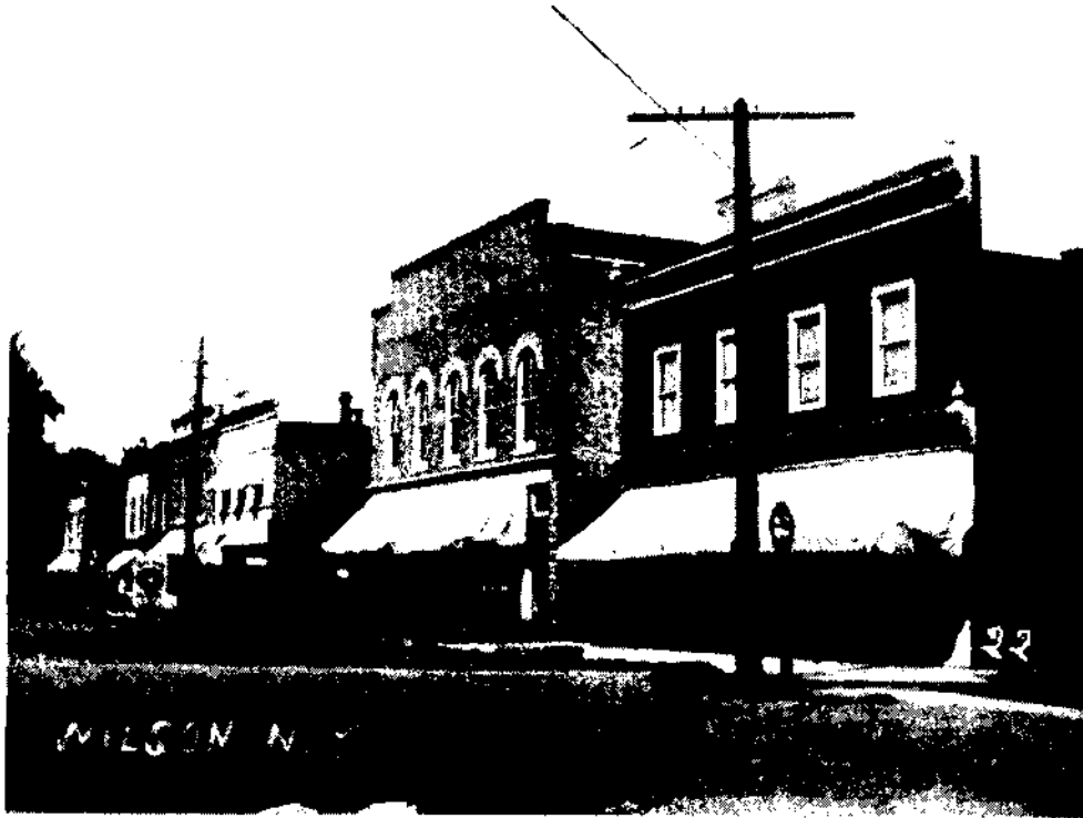
GAS LIGHT ERA, MILLER AND BROWN STORE ON CORNER
