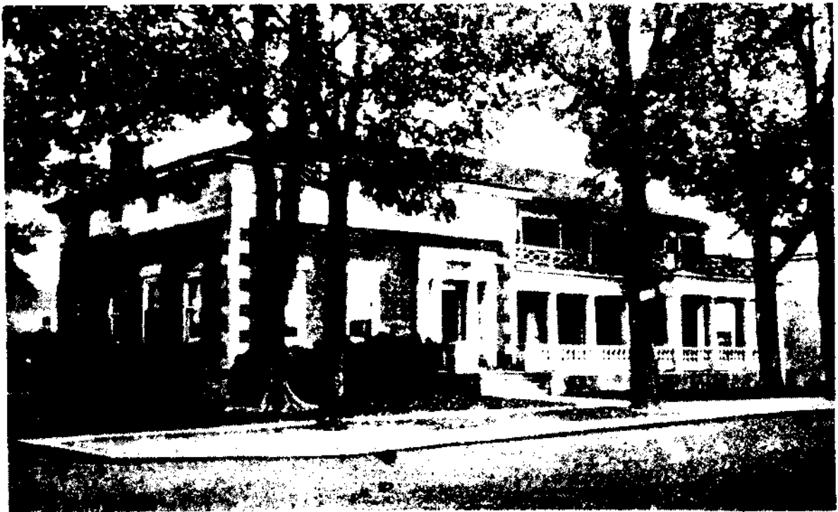
LUTHER AND REUBEN F. WILSON HOME Built in 1844 on site of first schoolhouse in Village
